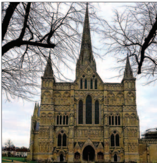
Salisbury Cathedral – Heritage high rise risk
