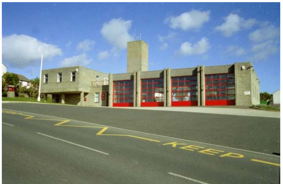
Newquay Fire Station
