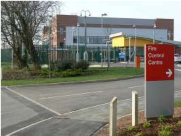
The South West RCC
